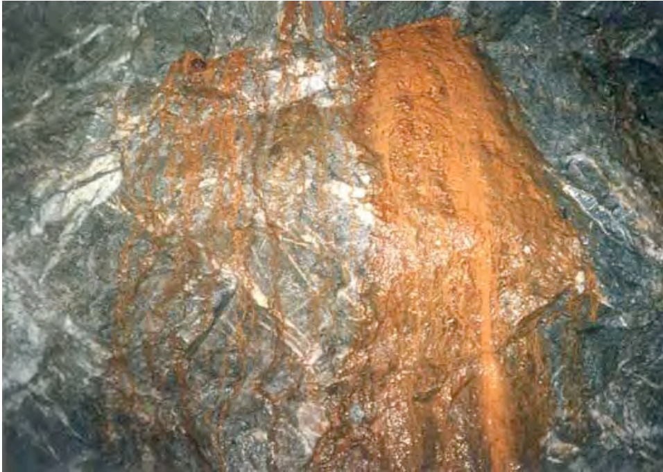
Figure 10: Acid Drainage photo. Acid drainage is red or orange because of the iron in it. Dissolved oxidized iron gives acid drainage its distinctive red color. These processes occur naturally, but are more extreme when rock is crushed and more rock surface is exposed. Acid on tunnel walls at Kensington gold mine (Southeast Alaska). Photo - D. Chambers.
