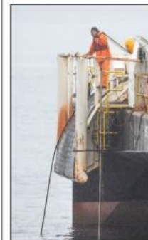
Above, a Westpark Electric crew moves between shore and barge on Thursday during installation of a fiber-optic cable at Mountain Point. The barge Empire 45 arrived early Thursday morning with tugs Arctic Tag and Island Tugger. Crews connected the cable from Prince Rupert to Ketchikan at a recently constructed communications hub at Mountain Point. Fiber-optic cable was unraveled from a large orange spool located at mid-ship and was fed off the stern of the barge.
