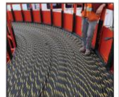
The submarine fiber-optic cable is shown spooled aboard the barge Empire 45.
