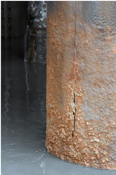
Cracked Pile
