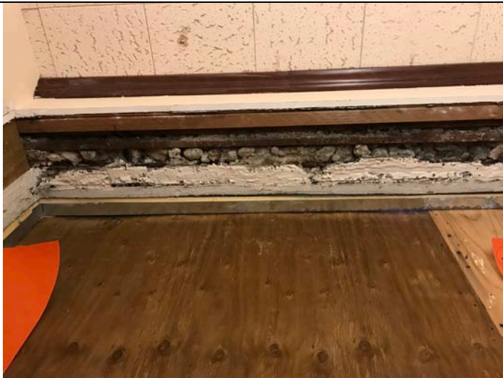
View of third floor heads.
