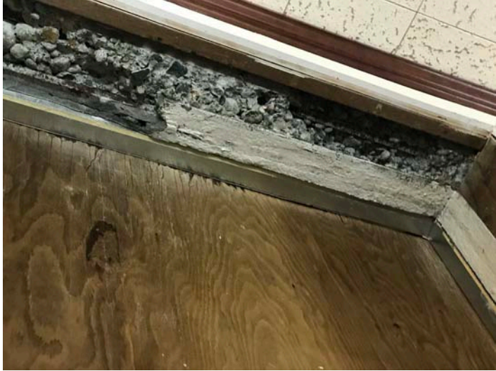
View of third floor heads.
