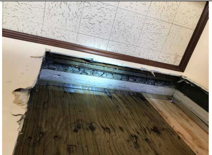
View of third floor heads.
