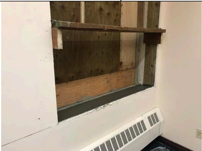
View of typical window sill grout repair.
