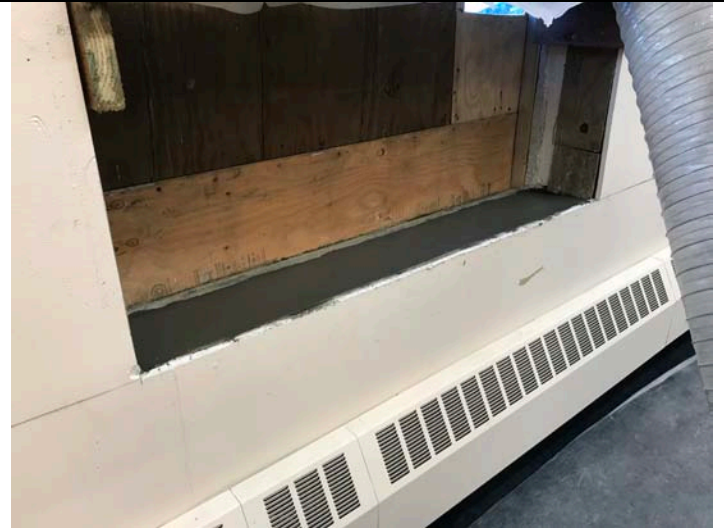
View of typical window sill grout repair.
