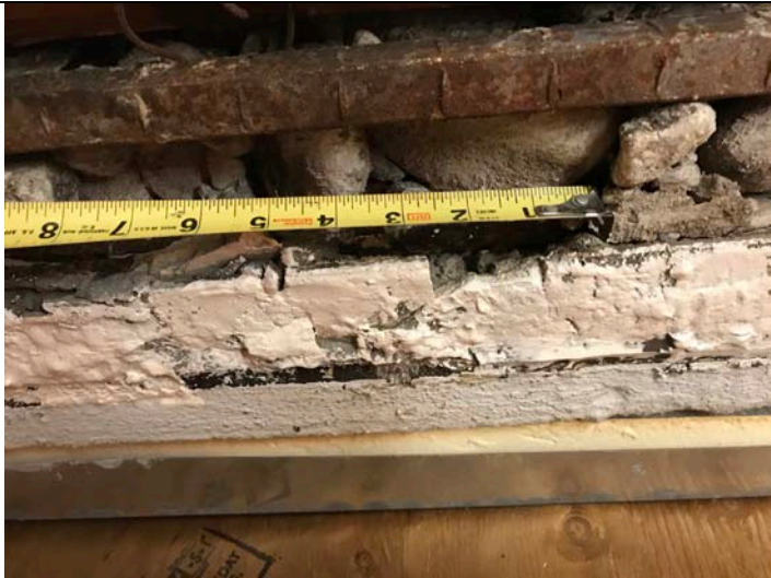
View of third floor heads.
