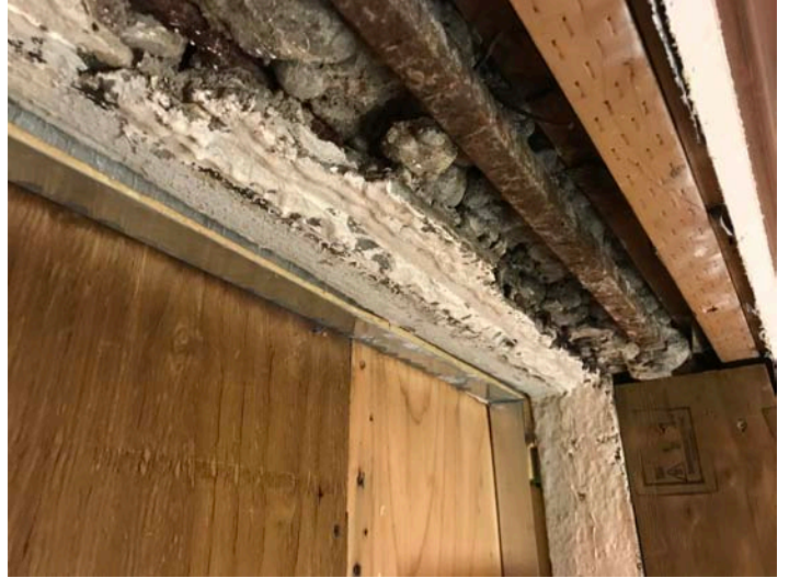
View of third floor heads.
