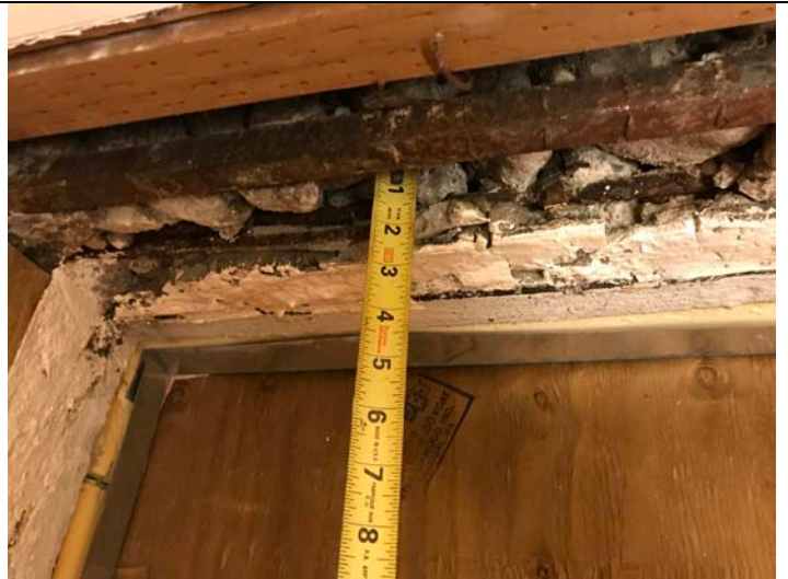
View of third floor heads.
