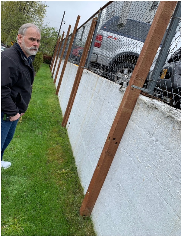
Temporary Fence Anchors
