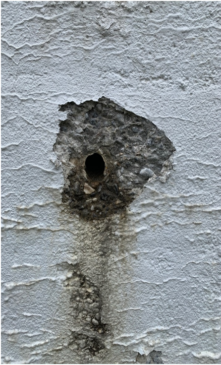
Existing Drain Holes
