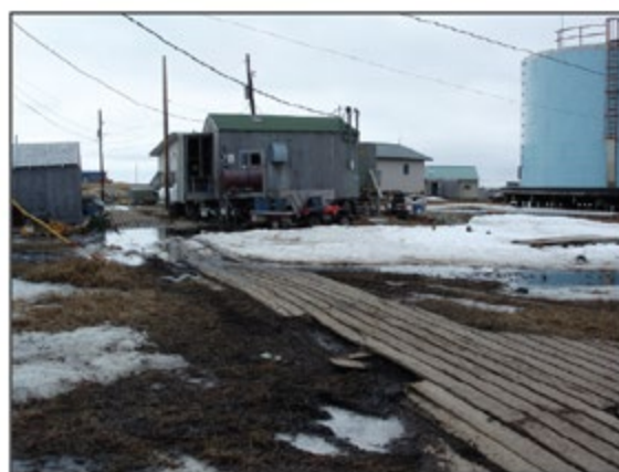
Figure 22.4. Residents in Newtok, Alaska are living with the effects of climate change, with thawing permafrost, tilting houses, sinking boardwalks, in conjunction with aging fuel tanks and other infrastructure that cannot be replaced because of laws that prevent public investment in flood-prone localities. (Photo credit: F. S. Chapin III).
