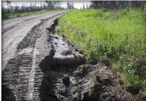
Failing Drainage
