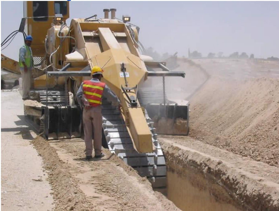
Figure 2. Chain Trencher
