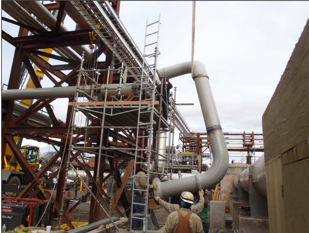
Recirculation pipe installation at PS4
