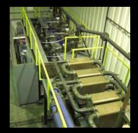
Improve the design, reduce the cost, and improve operation capacity of the **Chena Power Energy System**. This third generation system is modular, requires no foundation, produces 300 net kWh. It is synchronous and therefore requires no grid.
