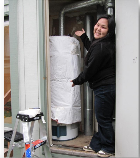
Installing water heater blankets and teaching maintenance
