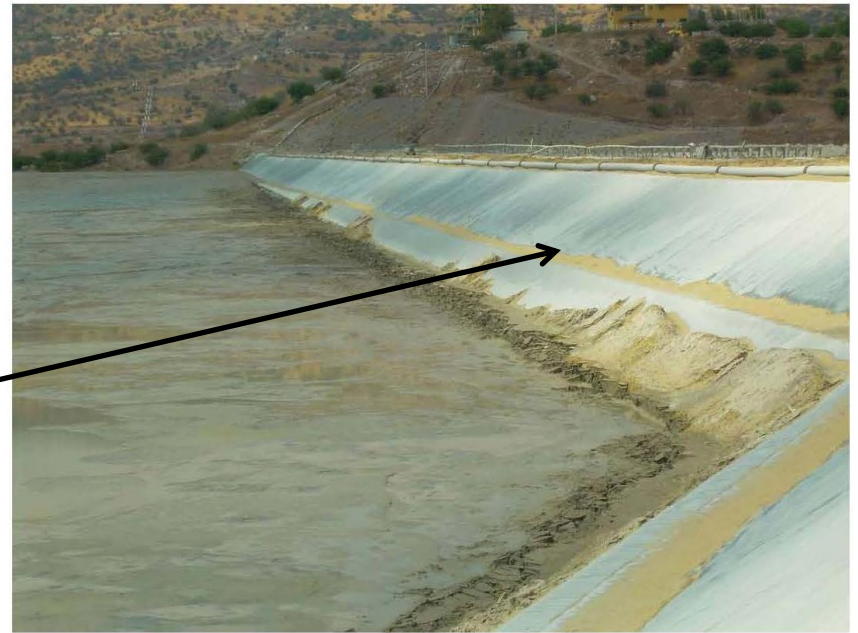
Figure 11.12. March 10, 2010. Upstream face of the Ovejeria Tailings Dam showing approximately 0.5 m of the tailings adjacent to the dam. (S33.052081, W70.792067)
