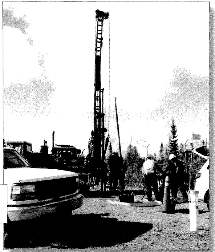
(Right) A Flint Hills contractor drills into the ground to install a new monitoring well, one of 80 installed this summer. (FHRA photo)
