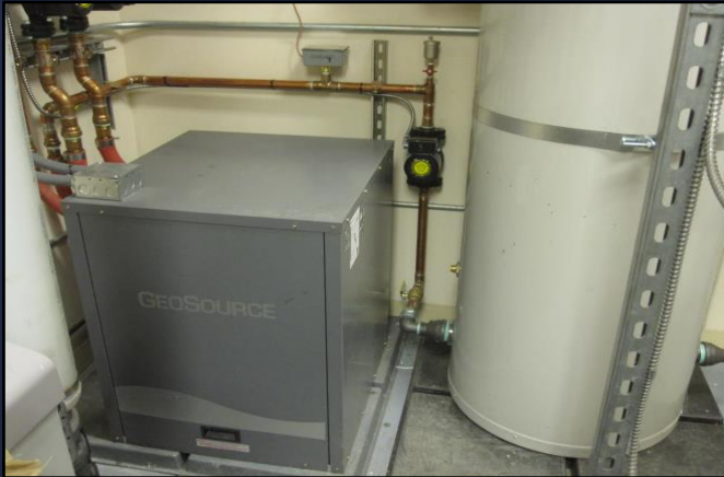
Installed 3-ton Heat Pump
