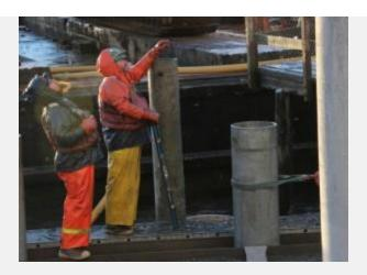
In between drilling, workers blow air into the piling to clear out cuttings and advance the drill, sending water and cuttings spitting out of the top of the piling. (KCAW photo/Rachel Waldholz)
