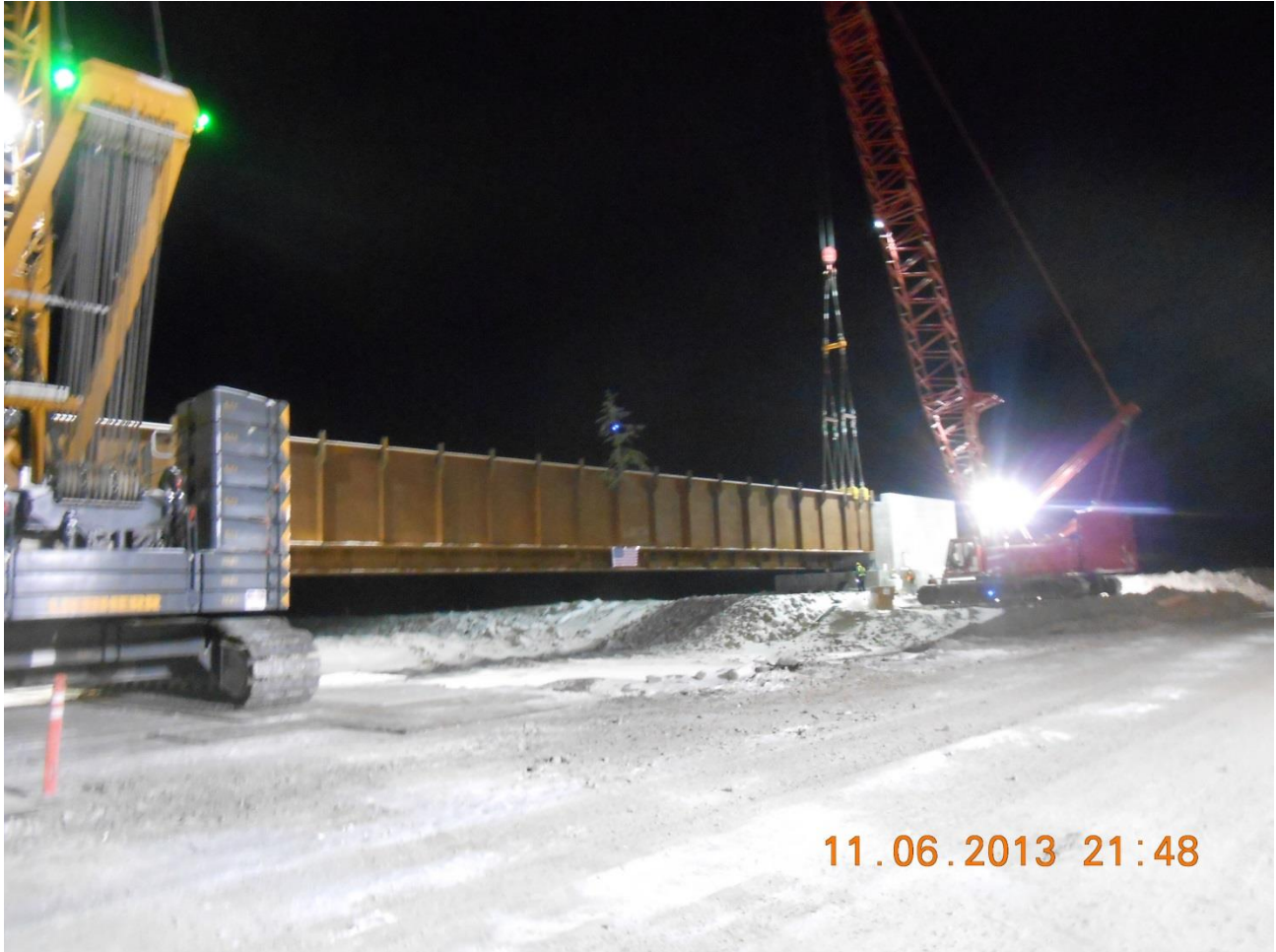
Last bridge girder erected
