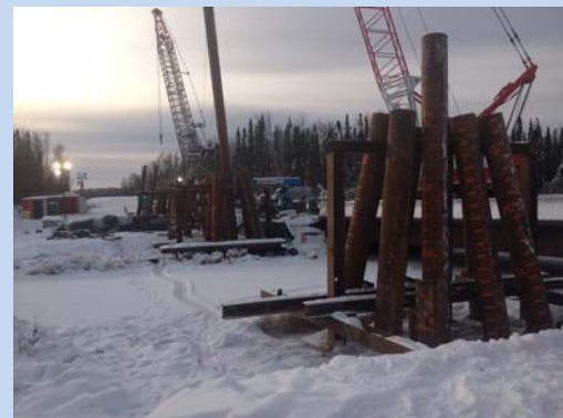
Driving Pile on Diamond Lake Outfall Bridge
