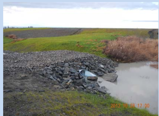
Drainage repair and improvements at BMBF pad
