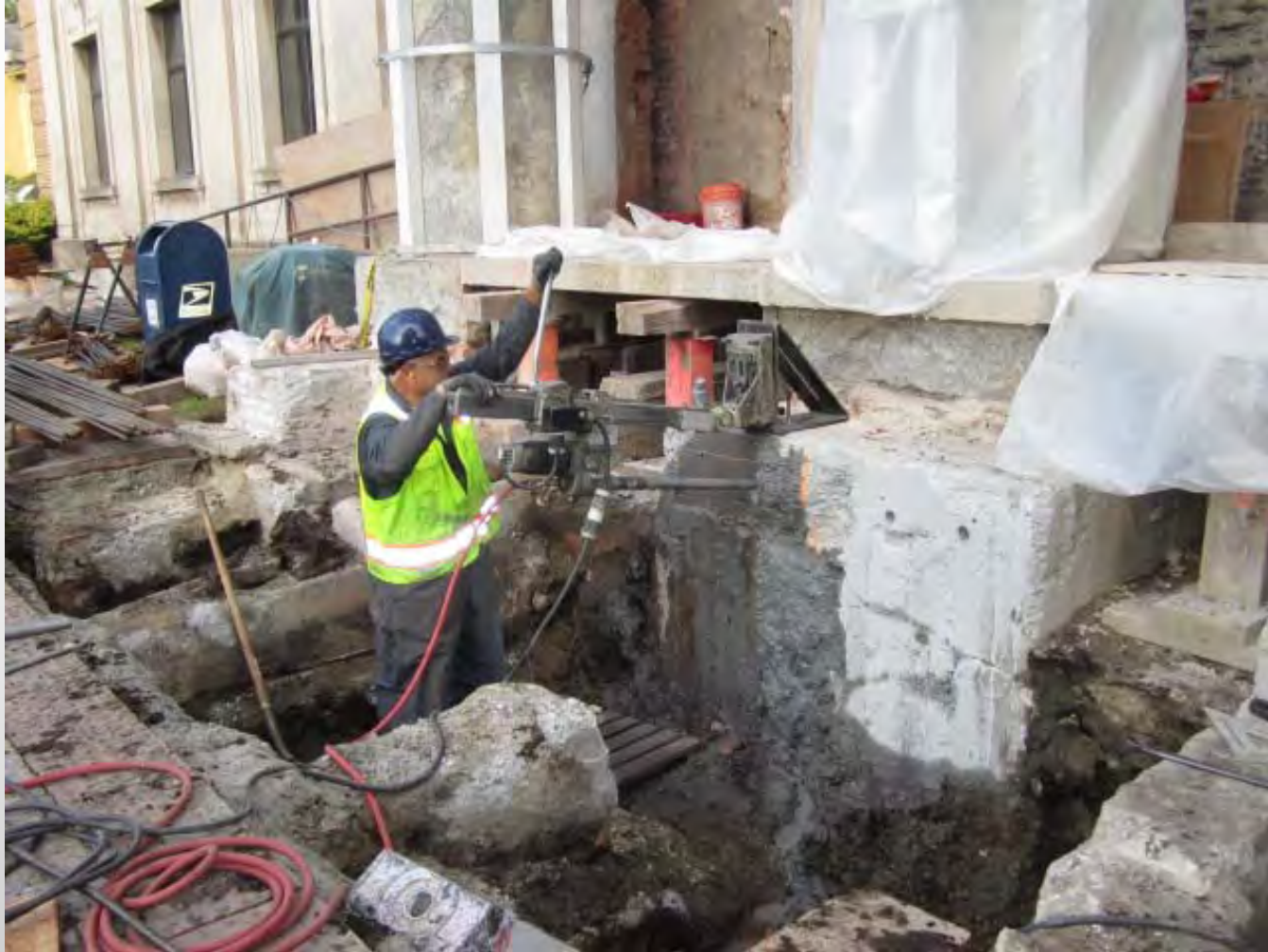
Drilling into Column Foundations for Reinforcing
