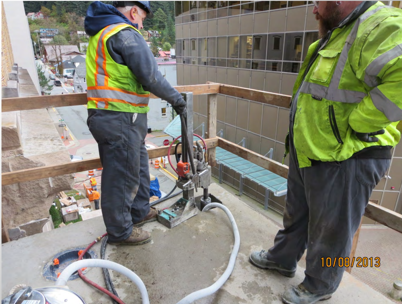
Core Drilling Columns for Reinforcing
