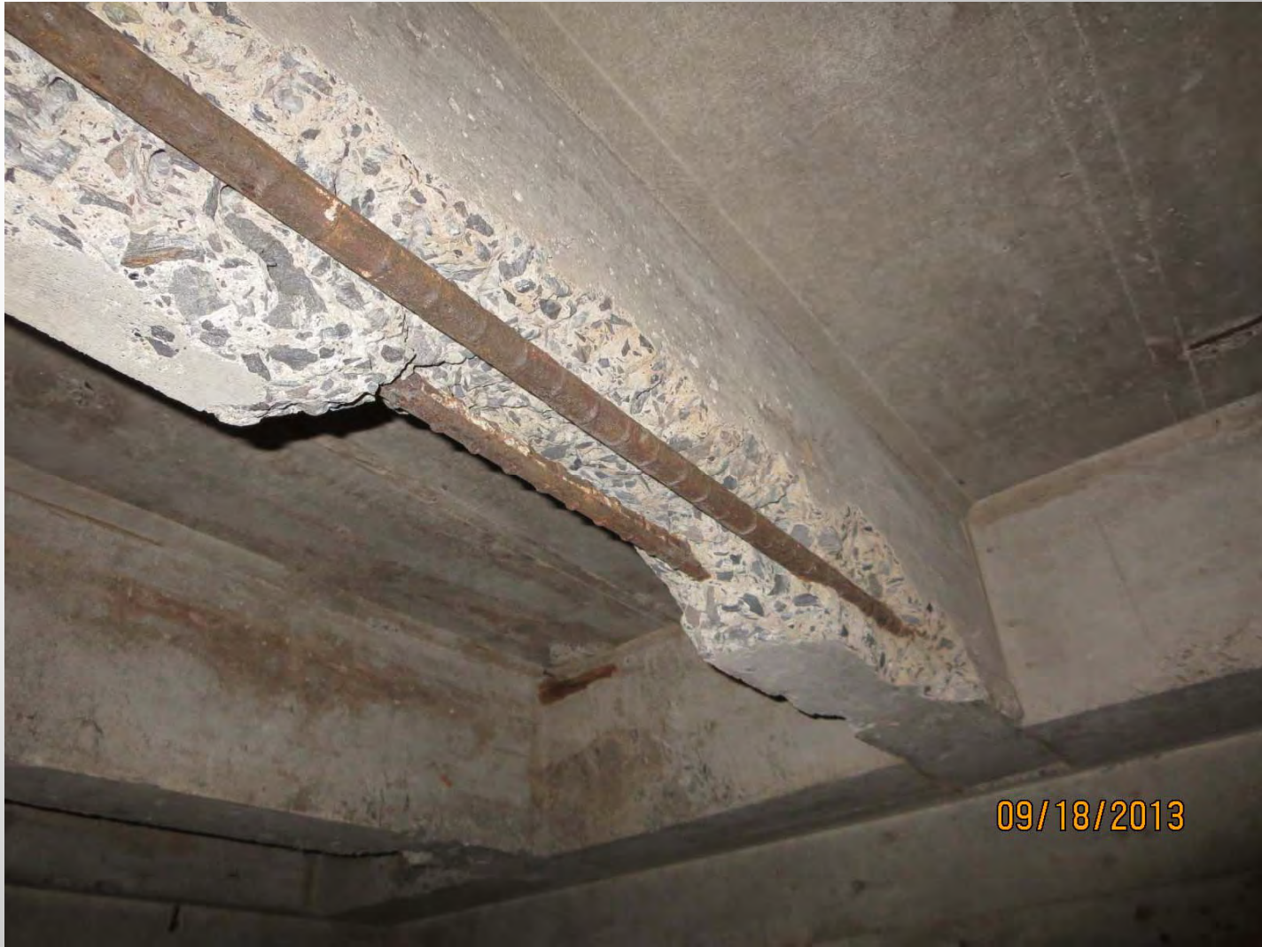
Loose Concrete and Rust removed from Joist
