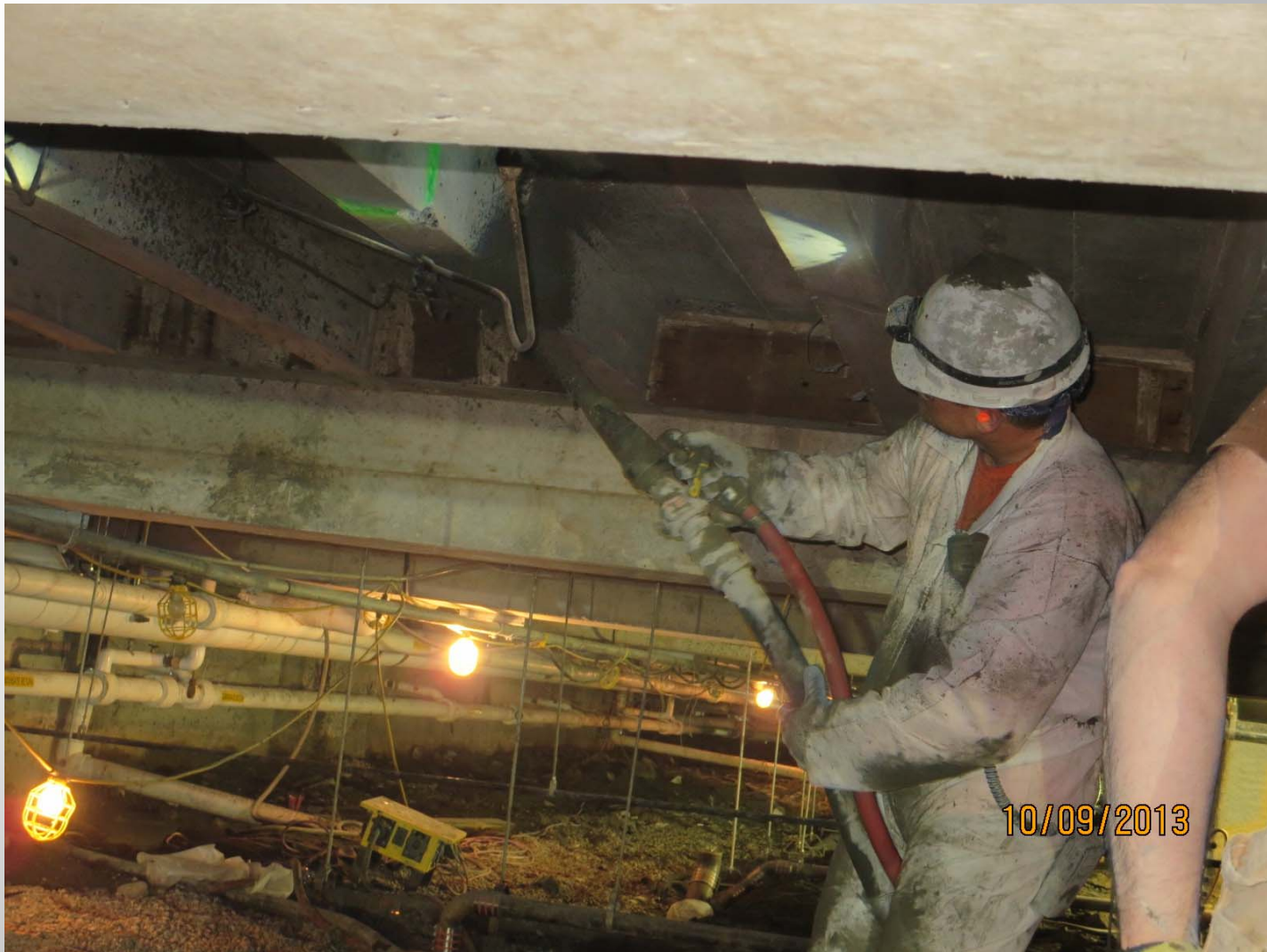
Shotcrete being Applied to Joists
