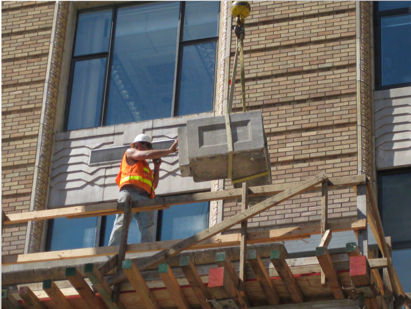
Stone being Removed from Portico Roof
