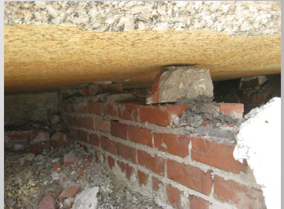
Condition of Foundation under Entry Stairs
