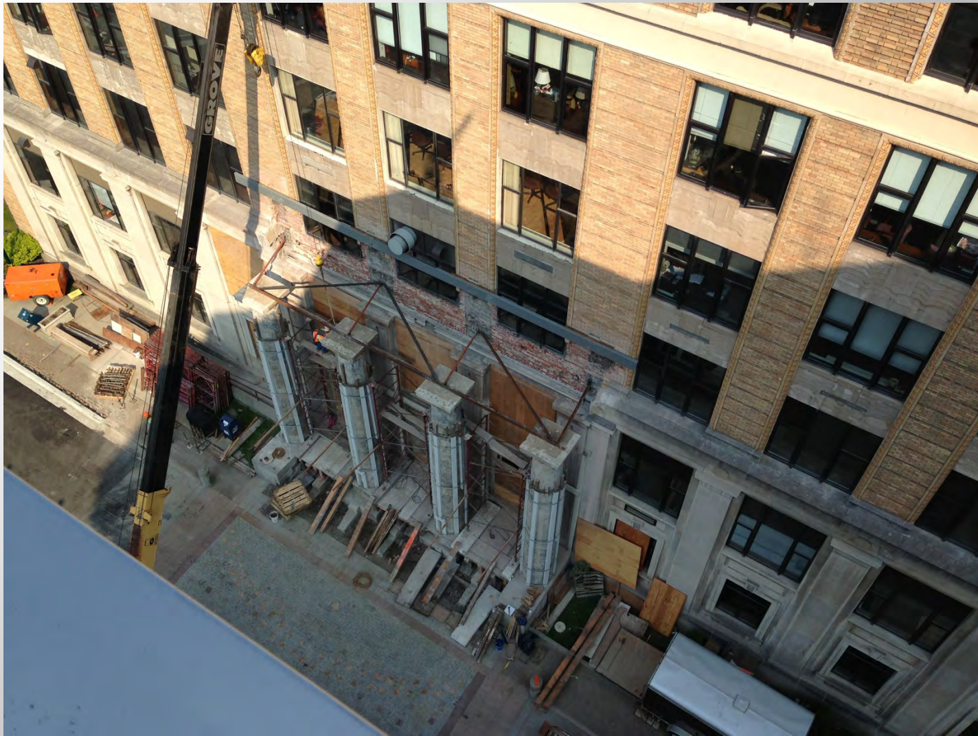
Stone Removed-Columns Braced
