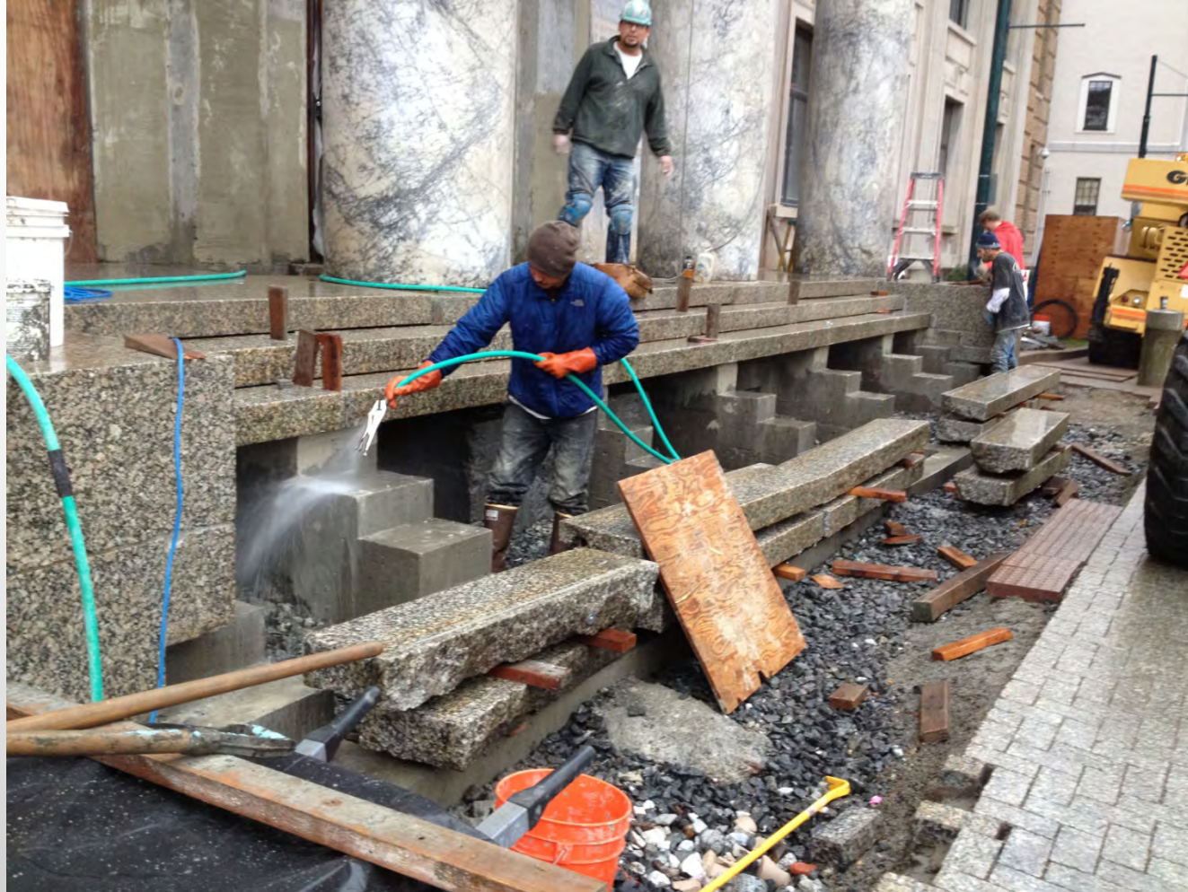
Granite Stairs being Installed
