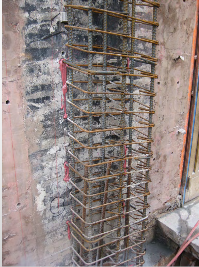
Reinforcing for Pilasters at Building
