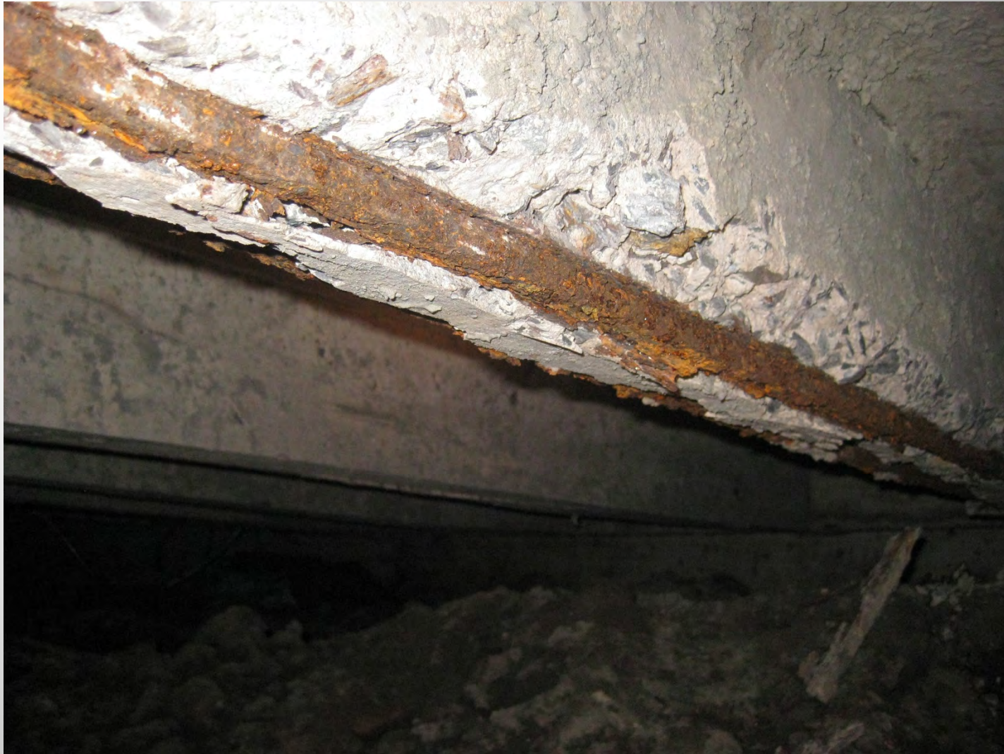
Corroded Reinforcing in Floor Joist
