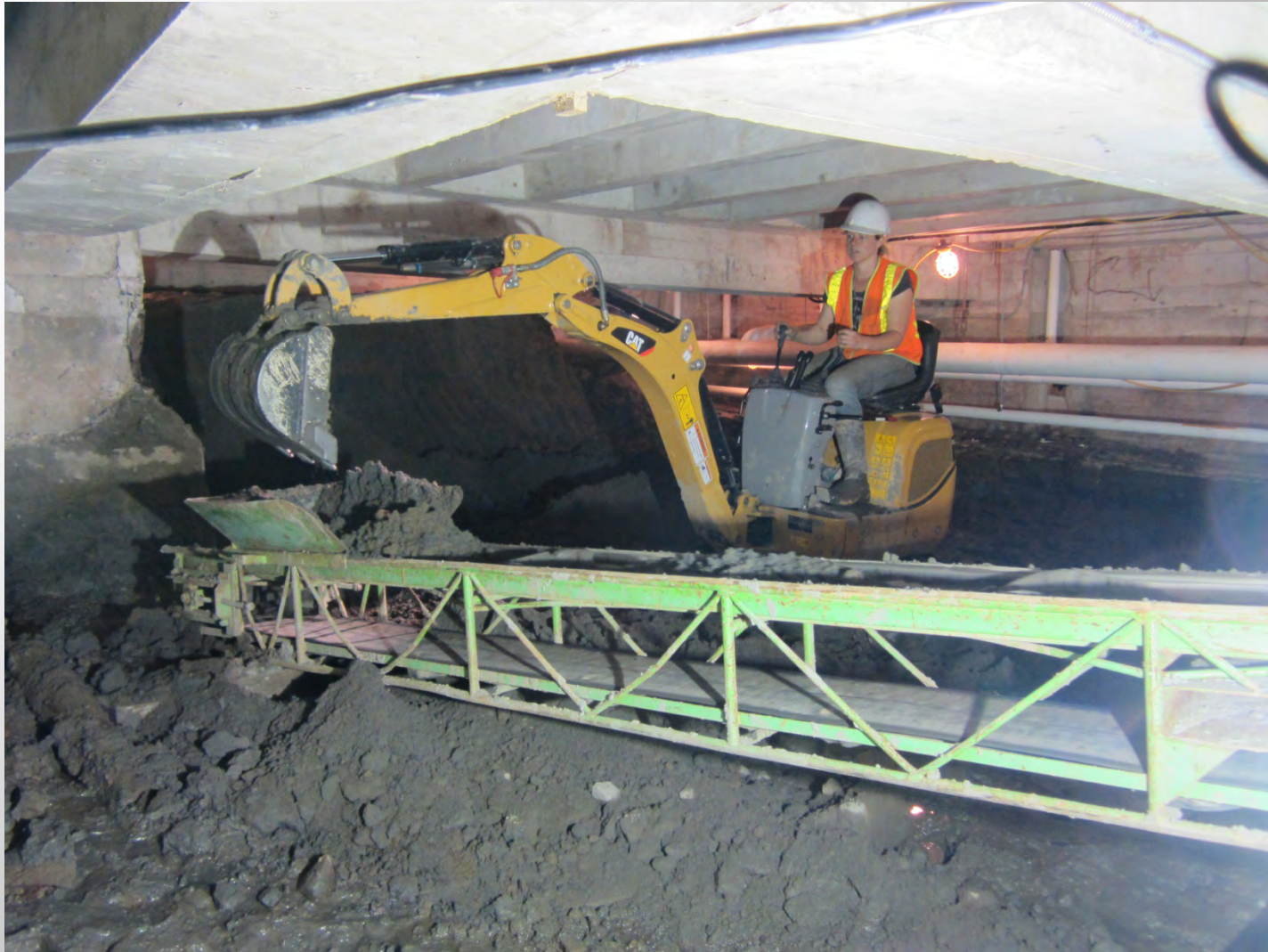
Removing Dirt from Crawl Space
