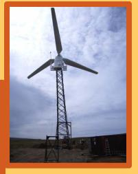
This specially designed tilt up tower eliminated the need for a crane.
