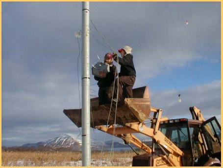
Raising the data logger to 25' in November 2005 prevented repeat damage. But attempts to install the predator proof fence around the tower (required by USFWS) were abandoned after persistent bear "intervention".
