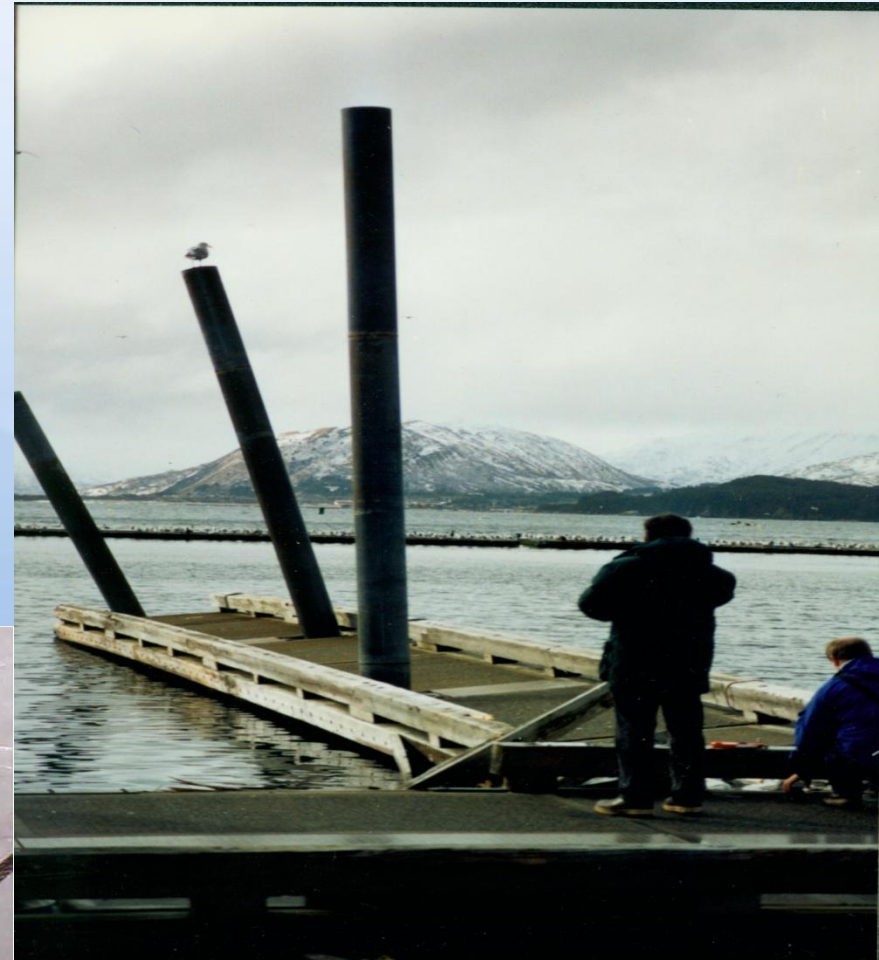
Bent piles at Kodiak
