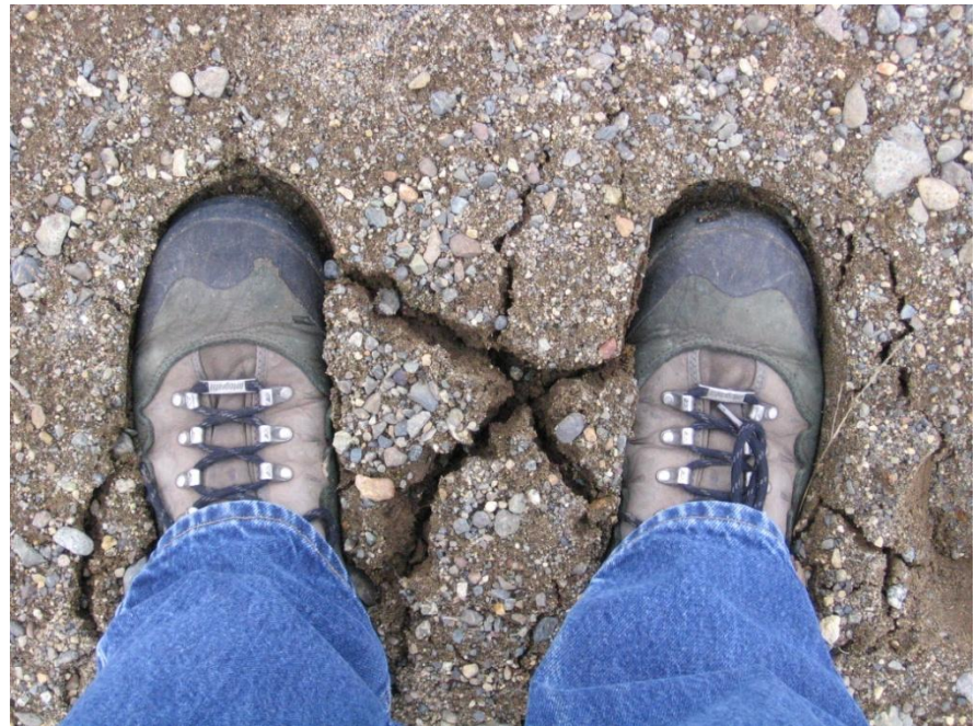
Soft runway surface at South Naknek Airport
