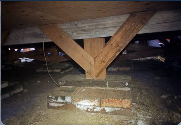
Typical Foundation Bracing (Kwigillinok)
