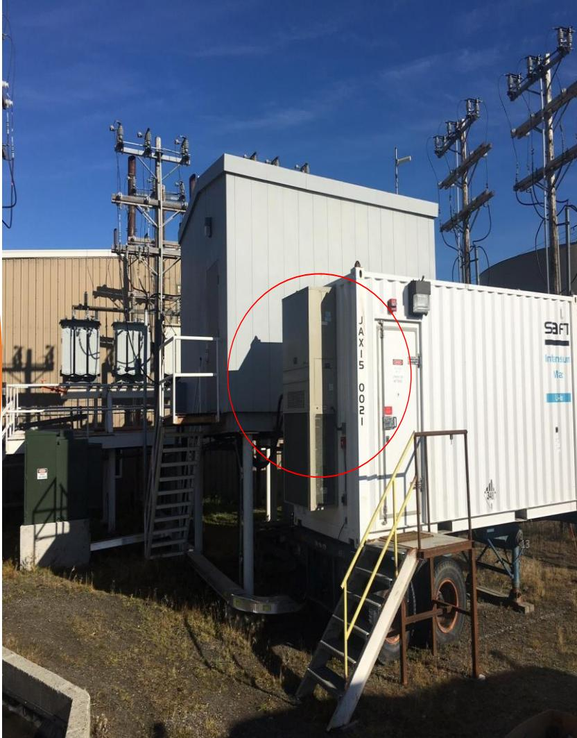
**Proposed 4MW 2MWh Battery**
