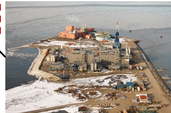
Oliktok Point Production Facility (OPP)
