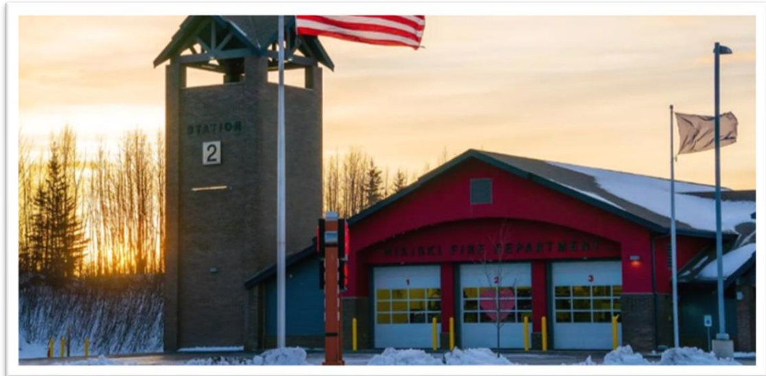
Nikiski Fire Department Station
