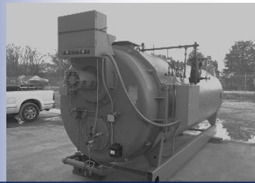
250 kW electric boiler as dispatchable load and saves diesel fuel 1500 gal/month
