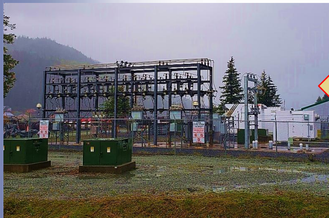
CEC Microgrid's Eyak Substation with BESS
