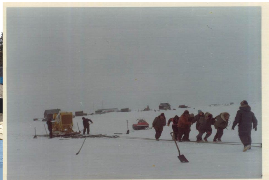
2. An 8000 lb. generating unit is placed upon a sled by block-and-tackle and manpower.
