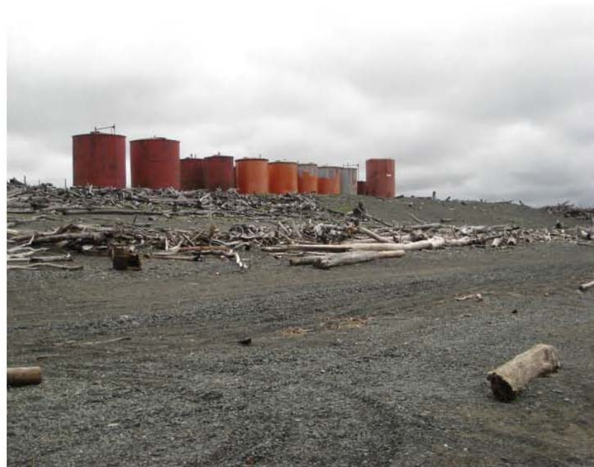
Photo 1: Shaktolik tank farm threatened by wave-driven driftwood and erosion
