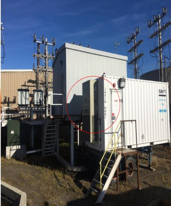
SAFT 950kWh Battery Container in Substation
