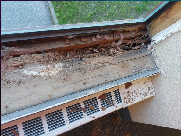
Weller Elementary Rotten window sill
