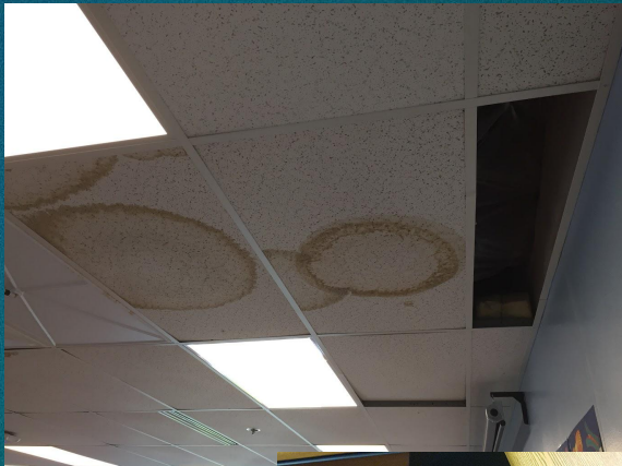
Arctic Light roof leak
