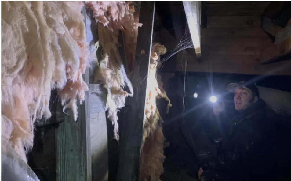
Taylor Hayden points out a series of wall studs underneath the school gym that aren't attached to anything anymore. Many are split down the middle. In 2021, an architect recommended Sleetmute's school be condemned. (Emily Schwing/KYUK)
