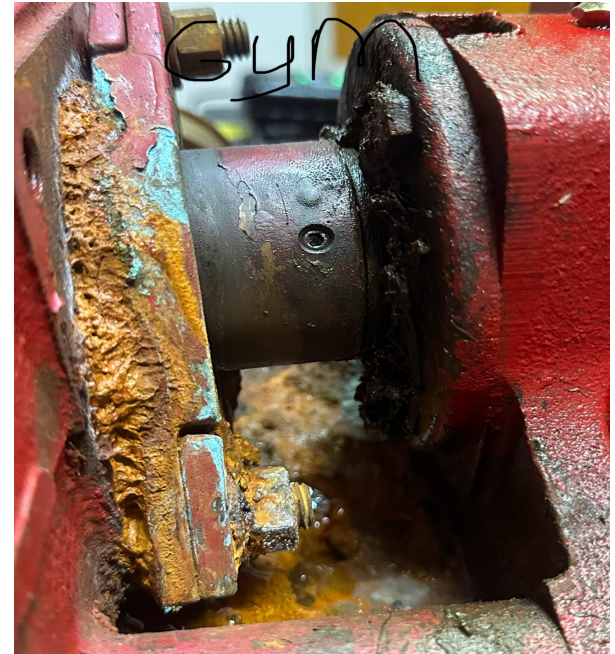
Thorne Bay School Fire Suppression System - Southeast Island School District - Project #38
