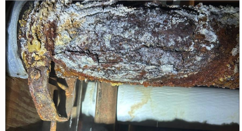
Residential Campus Hot Water Supply Pipe Corrosion
