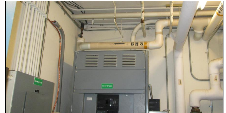
Electrical Panel exposed to aging pipe systems leads to failure and disruption to operations
