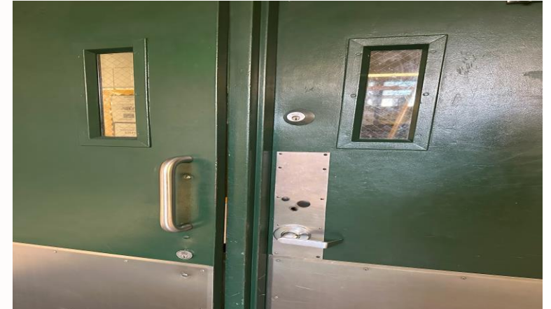
Avis Alaska Sports Complex – Door Hardware Failure
