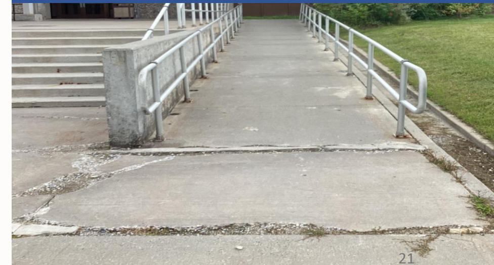
Broken/Uneven concrete preventing ADA Access up ramp
