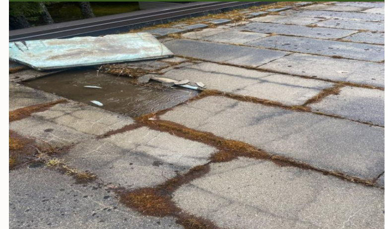
Campus Center Roof and Saturated Insulation
