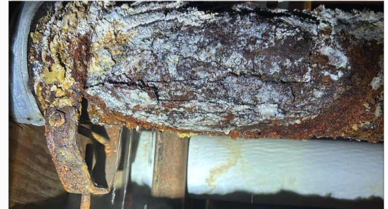
Residential Campus Hot Water Supply Pipe Corrosion
