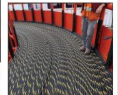
The submarine fiber-optic cable is shown aboard the barge Empire 45.
