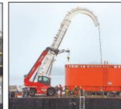
Above, cable is unraveled from a large spool, located topside at mid-ship, before being fed off the stern of the barge and onto the seabed.
