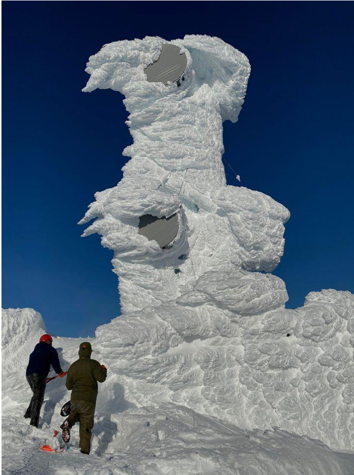
Alaska Power & Telephone Microwave Tower, Turn Mountain
