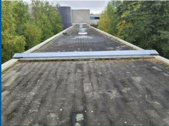
Roof & Seismic Joint
