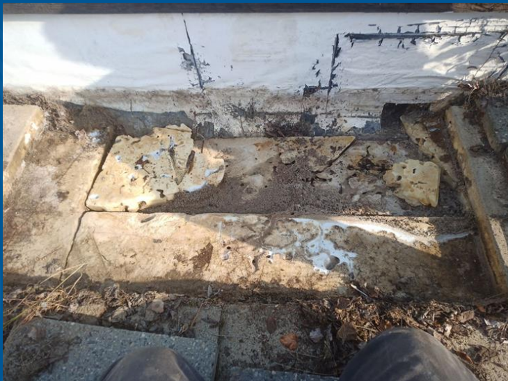
Cutler Housing Roof Failure
