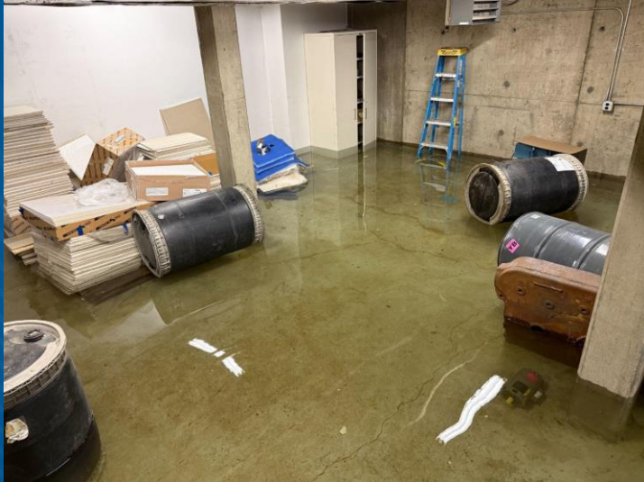
Valve Failure & Flood
