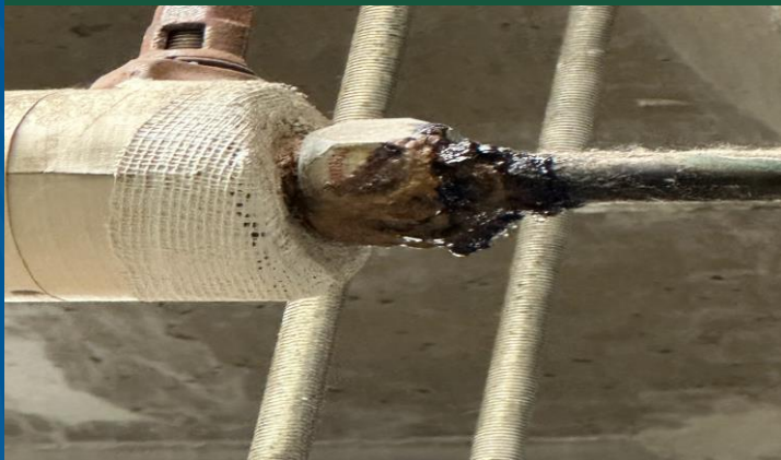
Boiler Leak
