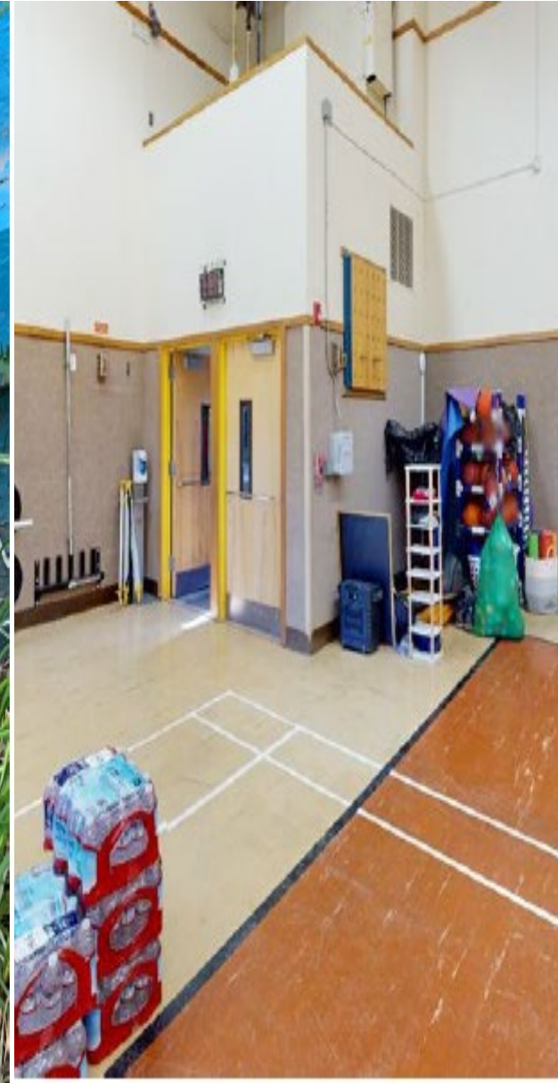
Multi-Purpose Room – A Project currently on School Construction List
