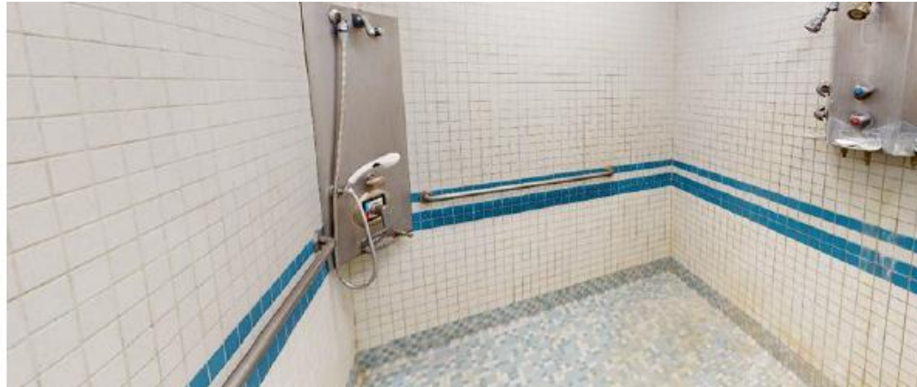
Boys Restroom – A Project currently on School Construction List
