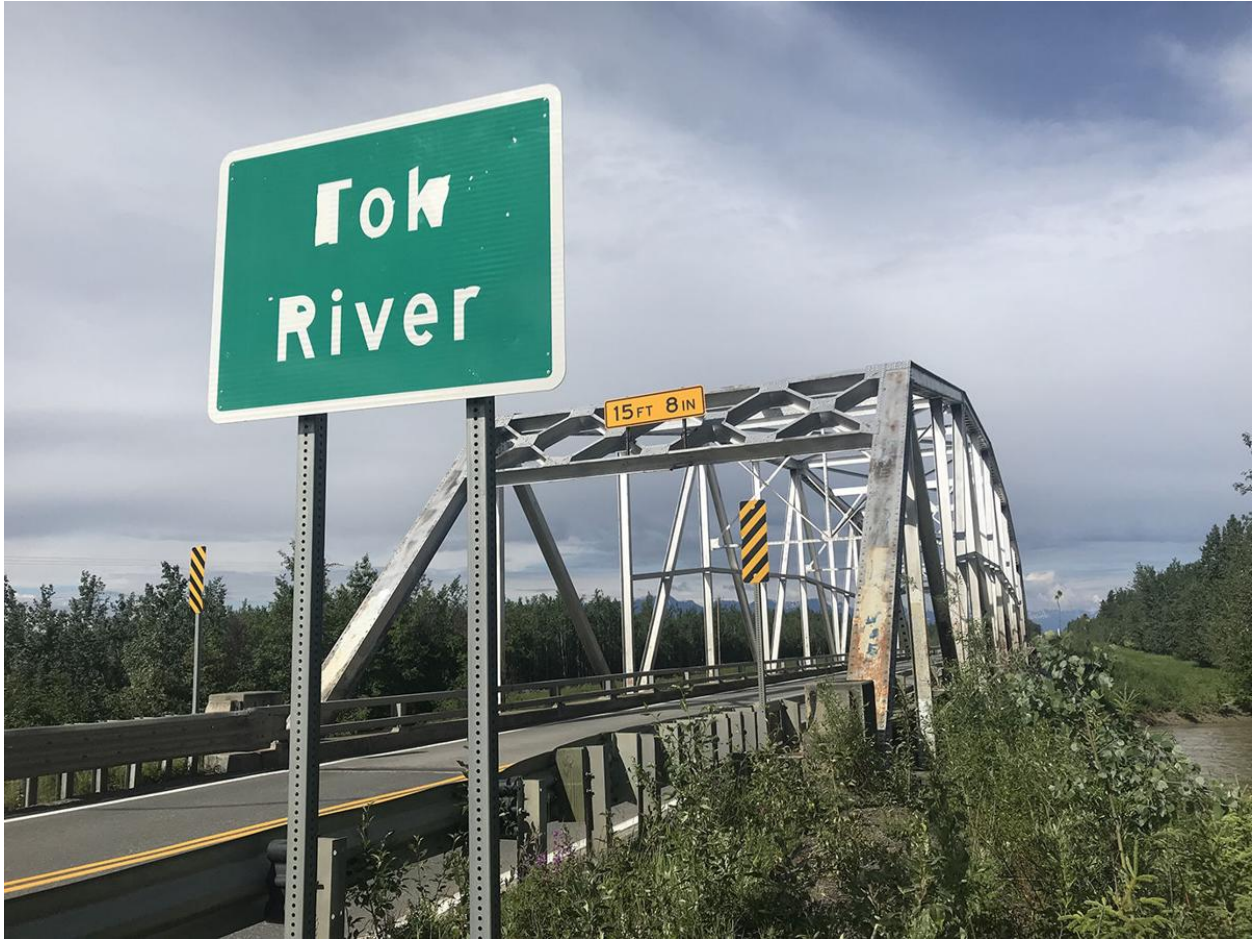
Old Tok River Bridge.
