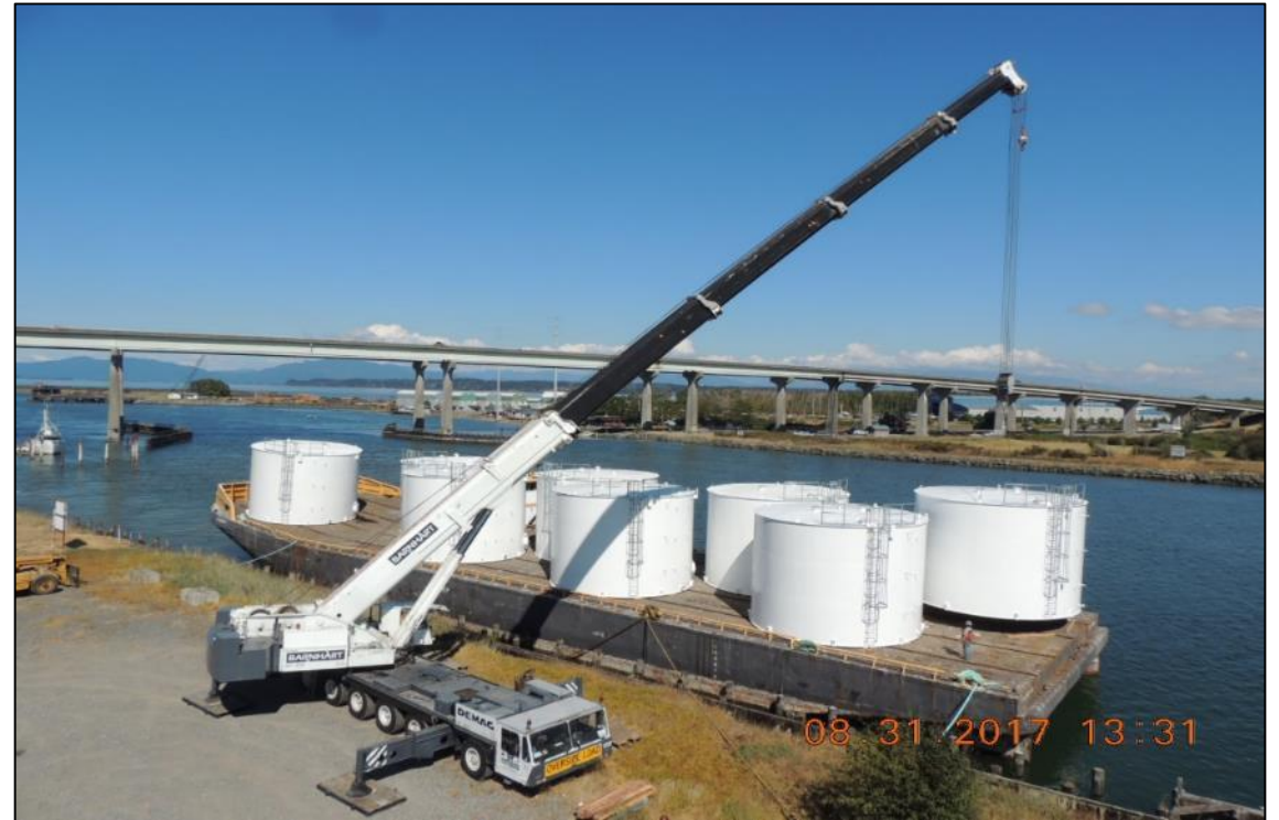
Kipnuk Bulk Fuel Tanks being loaded onto the barge in WA
