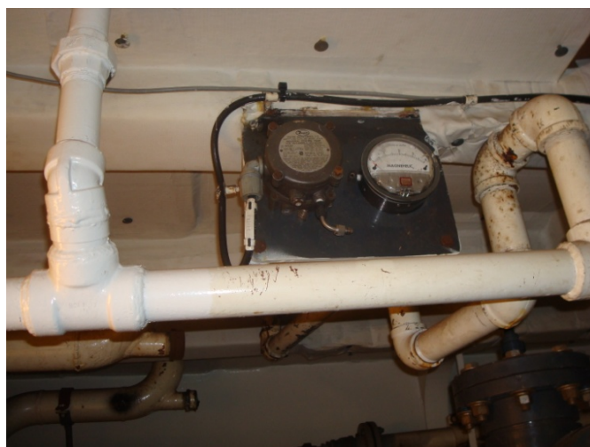
Photo 6-4 : Non Operational Port Vacuum Sensor and Gauge
