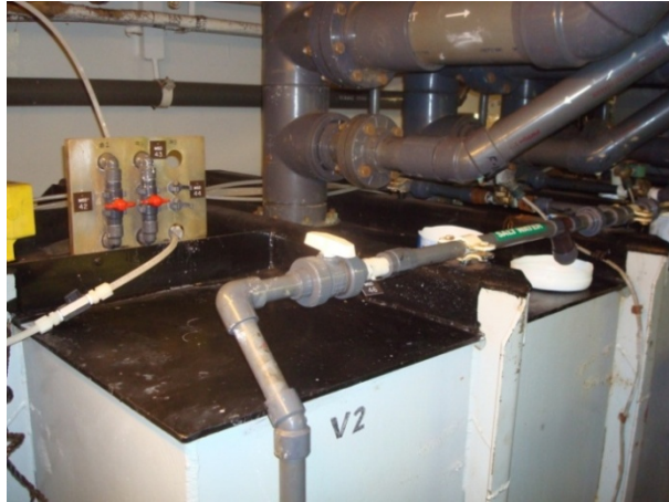
Photo 6-2 : External Chlorine Injection Distribution Manifold
