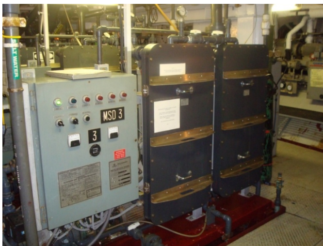
Photo 7-1 : Skid Mounted Single Pass 12MX bookcells and Control panel
