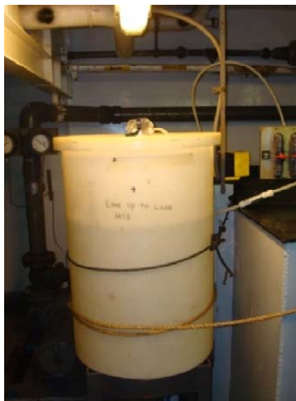
Photo 6-1 : External Chlorine Injection Tank
