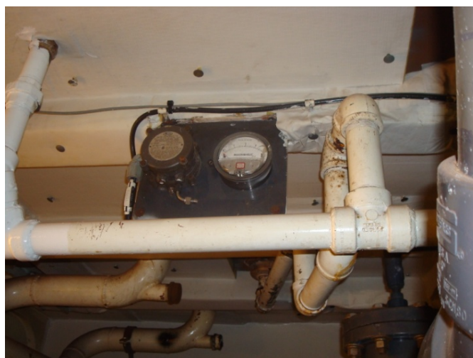
Photo 6-3: Non Operational Center Vacuum Sensor and Gauge
