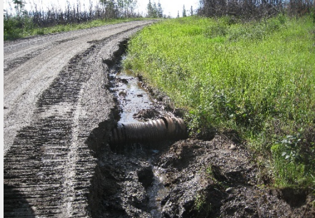
Failing Drainage
