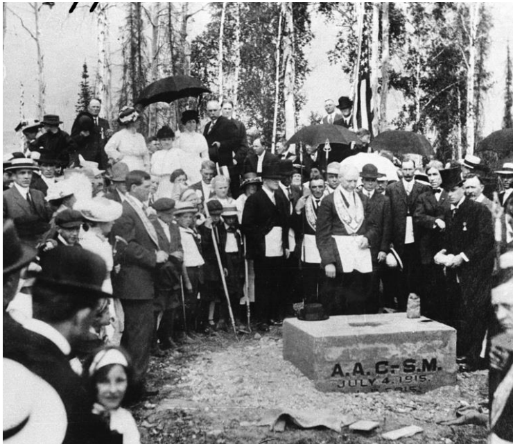
July 1915 - Laying the Cornerstone
