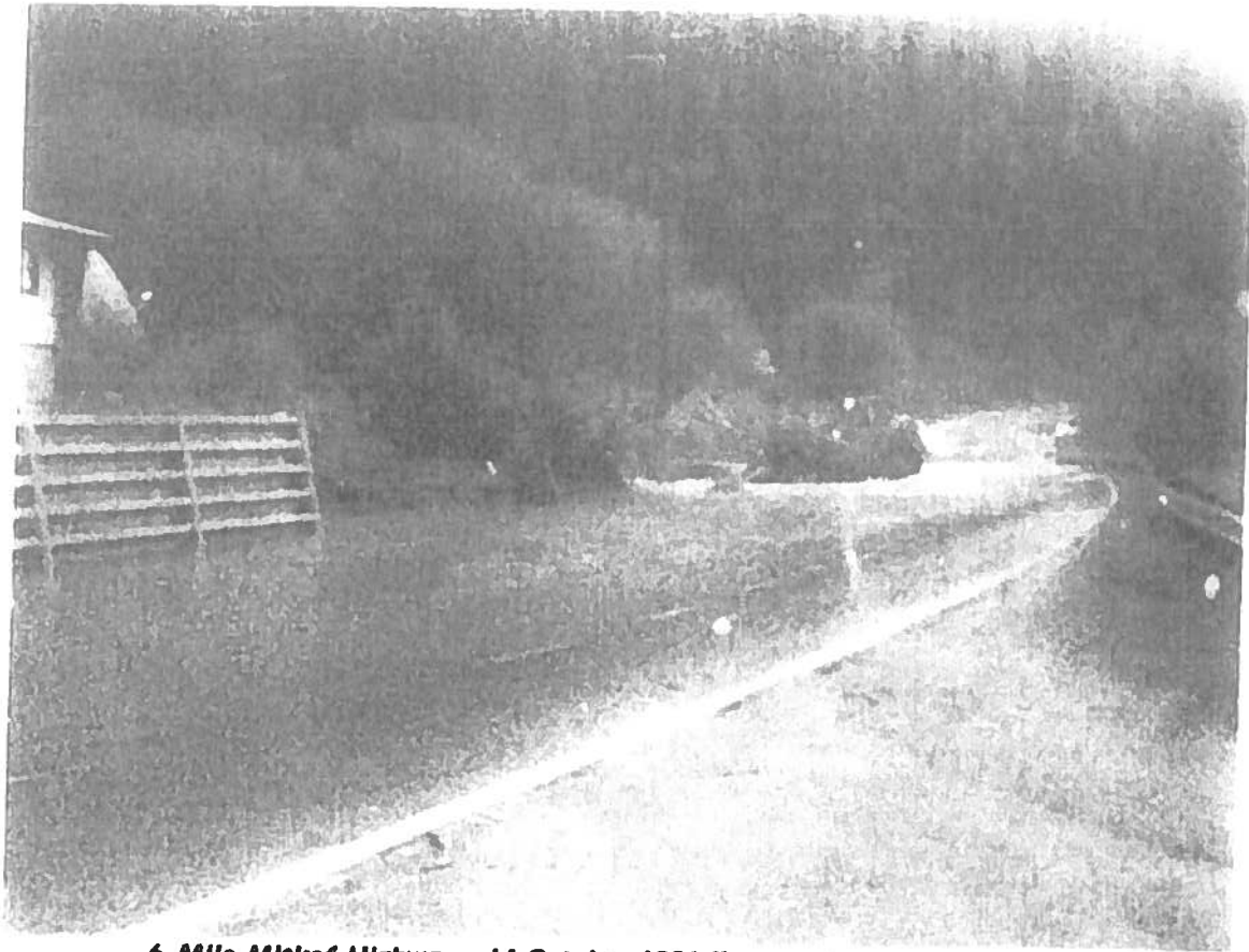
6-Mile Mitkof Highway - 14 October 1986 "natural" slide. This slide event originated at approximate 1400-foot elevation on Trust property. Alaska Department of Transportation workers are removing boulders, cobbles and organic material from the two culverts in Taain Creek to release flood waters and drain Mitkof Highway (State Highway #7) which was closed to through traffic. Bud/Judy Peterson's residential property is visible at photo and was impacted by slide. Dave/Kelly Peterson's home was not built at this time but the driveway at photo right bottom now leads to their home. Aaron/Katrina Miller now live at the other end of the guardrail on the downhill side. The Jones' family lives just past the DOT vehicles.
