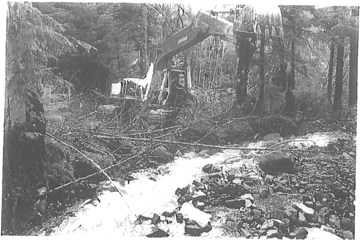
6-Mile, 1988 slide - Taain Creek cleanup and bank reconstruction. The 30 November 1988 slide that originated on Trust land at 1400 foot elevation coursed downslope with organic debris, and unmarketable harvested logs from a private property owner's clearcut timber harvest. The combination of the upslope organic debris, the unmarketable logs, and the runoff jumped the banks of Taain Creek impacting Bud Peterson's residential property at 6-Mile and onto Mitkof Highway, eventually spilling out into the Wrangell Narrows . During early Spring of 1990, the logging company contracted to have the unmarketable logs, boulders and organic debris removed from the lower portion of Taain Creek . The volume of debris in total required the rebuilding of the creek banks to an approximate 5-foot height.
