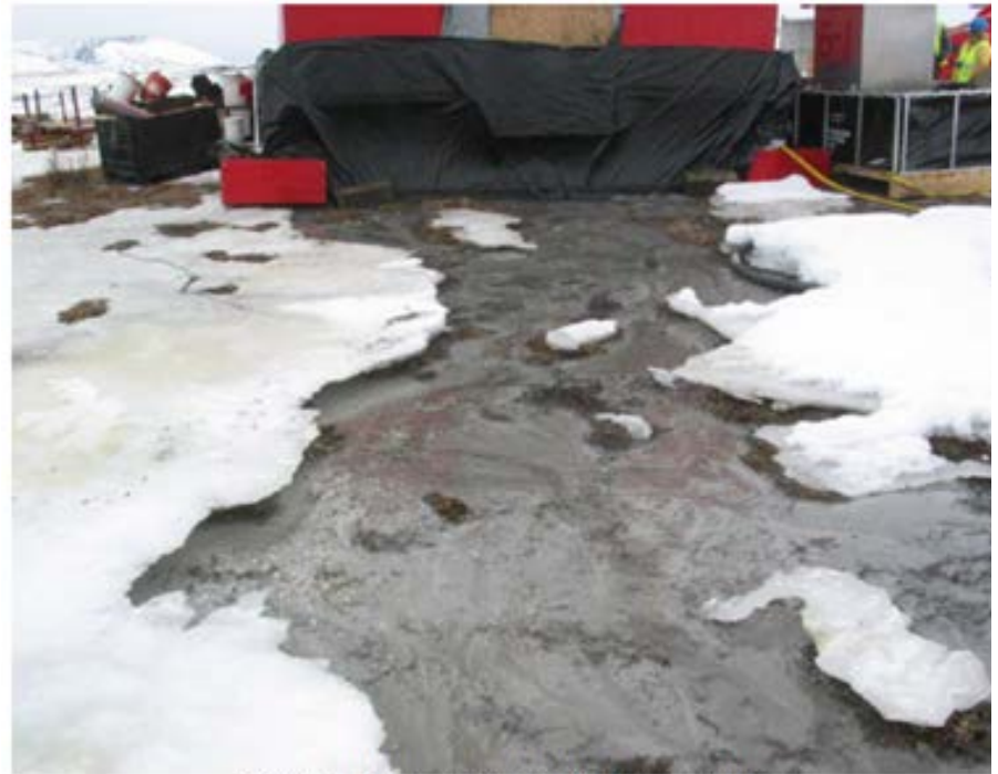
Figure 4. Water and cuttings discharge on uplands.
