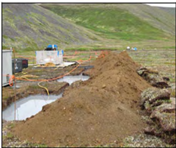
Figure 3. Sump pits (on left) and tundra stock pile being saved for reclamation (on right).
