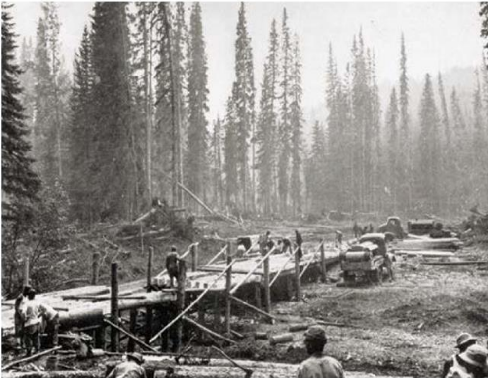
Black engineers build a trestle bridge during the construction of the Alaska Canada Military Highway. Black G.I.s made up roughly forty percent of the estimated 11,500 Army troops who in just nine months completed a wilderness highway linking Alaska with the contiguous United States.
