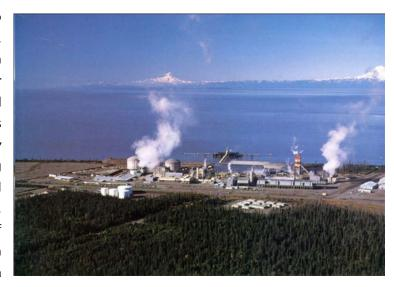
Operating at 50 percent of capacity, the operation will consume approximately 75 to 80 million cubic feet of gas per day (75 to 80 mmcf/day) or about 26 to 28 billion cubic feet annually (bcf/year). It will produce 630,000 metric tons of ammonia (about half or which is used in the production of urea) and 620,000 metric tons of urea. With both trains in operation, gas consumption and production of ammonia and urea would be double these amounts.
