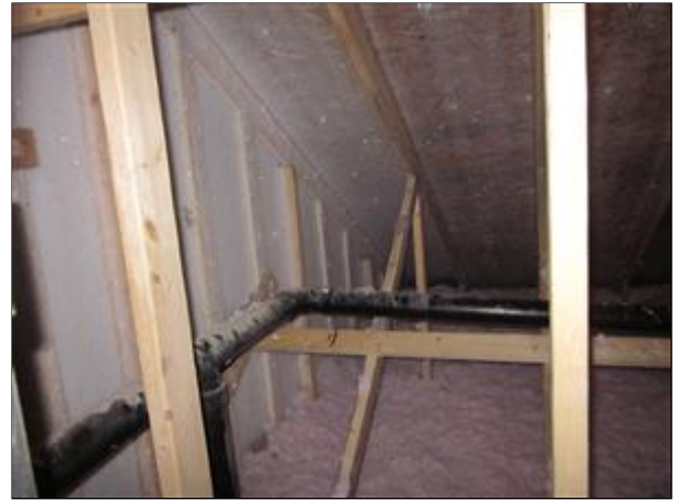
8.3 Picture 6 Frost buildup on interior of gable end in attic
