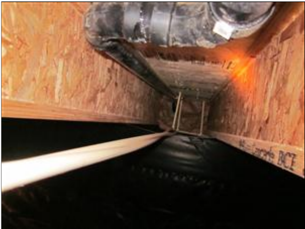
5.0 Picture 6 No vent within required distance of fixture
