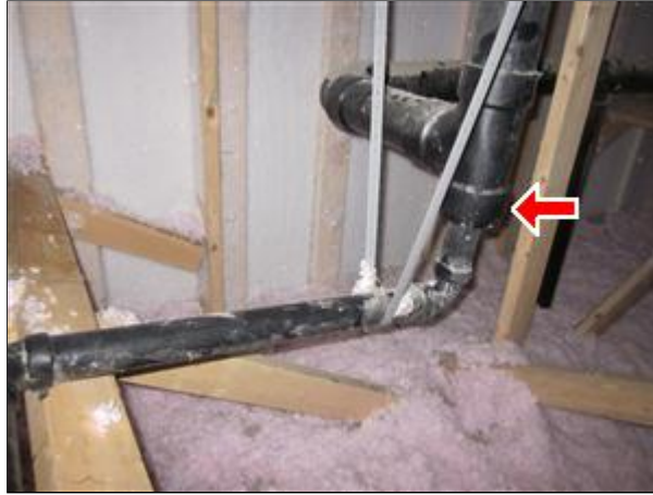
5.0 Picture 7 Less than 2" vent pipe is undersize, and change in vent size not made in insulated space as required.
