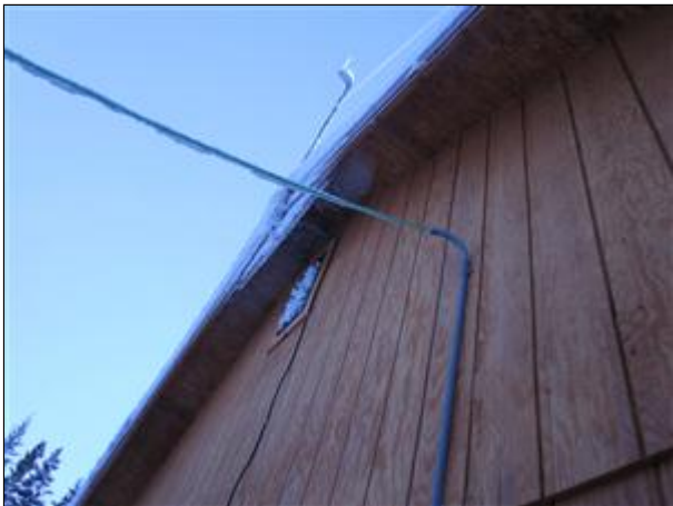
8.3 Picture 1 Frost exiting gable end vent
