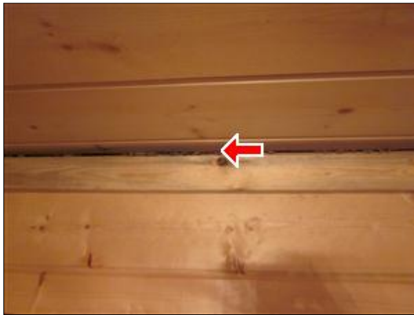
8.3 Picture 7 Attic insulation visible from inside of master bedroom, trim piece falling down.
