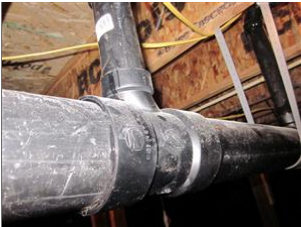
5.0 Picture 2 Improper fitting
