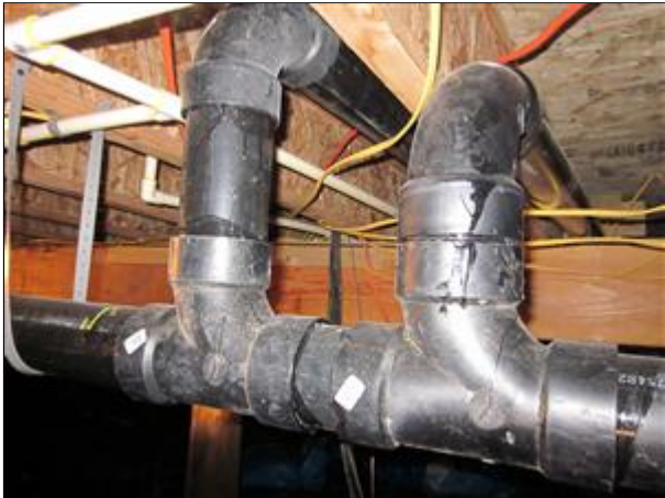
5.0 Picture 3 Improper fittings
