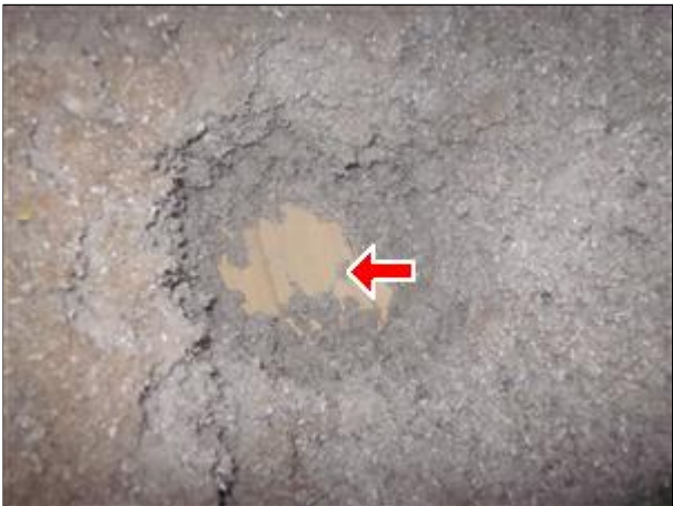
8.3 Picture 2 no vapor retarder over ceiling, under insulation.
