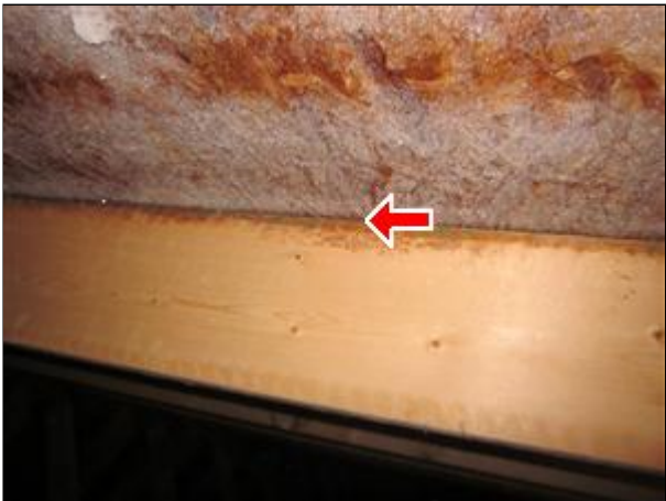
8.3 Picture 4 Beginning moisture damage at top of truss and roof sheathing.
