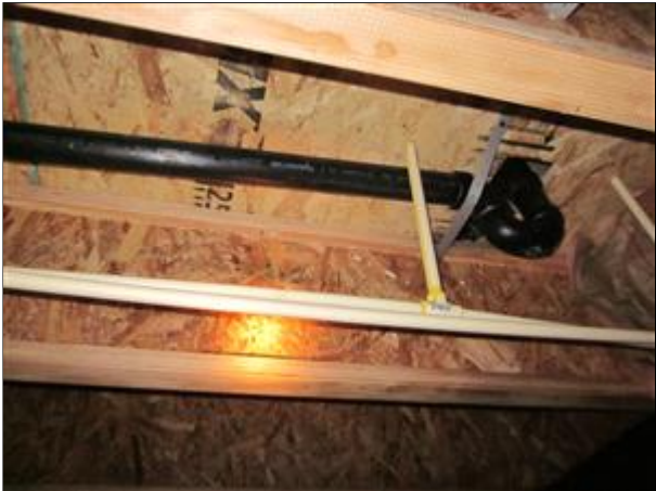
5.0 Picture 4 Incorrect fixture venting
