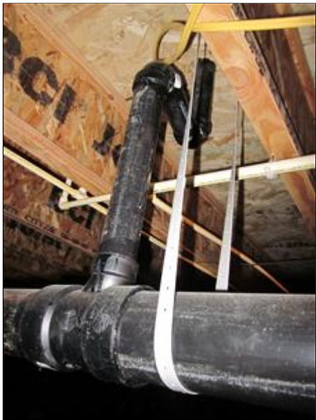
5.0 Picture 1 Improper fitting
