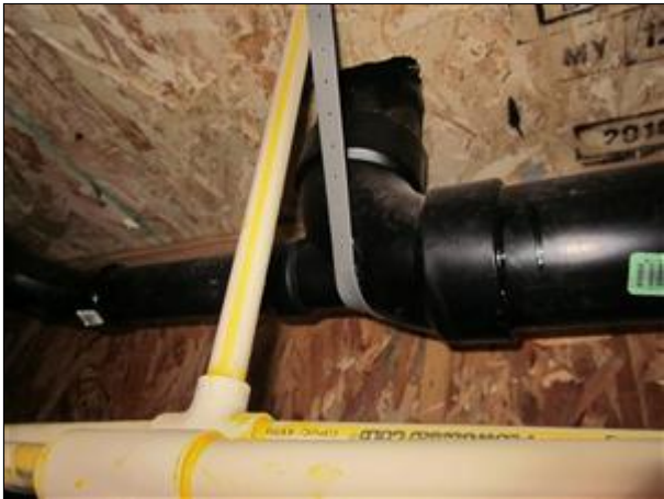
5.0 Picture 5 Incorrect venting
