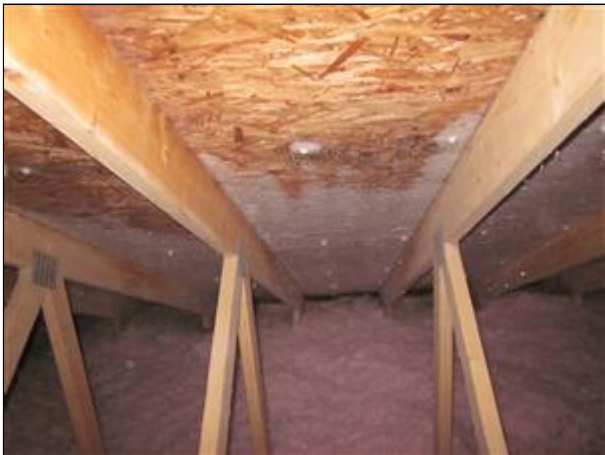
8.3 Picture 3 Frost buildup on roof sheathing.
