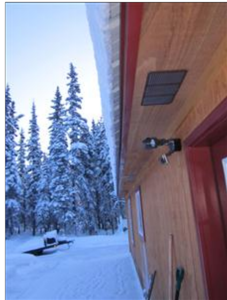
8.3 Picture 8 Soffit ventilation at rear of house.
