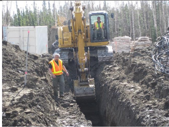
Digging the trench for the coil
