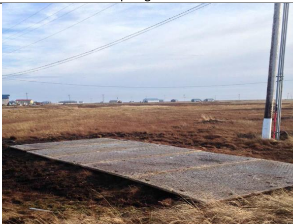
Site mats positioned awaiting the battery
