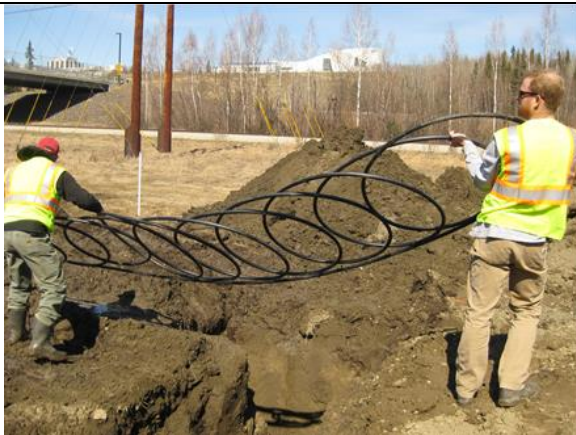
Installation of the slinky loop
