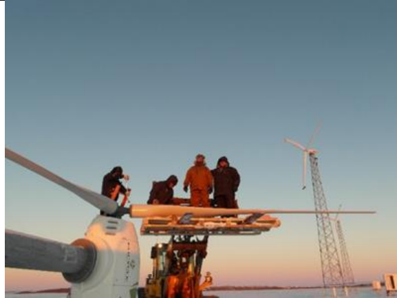
Installing turbine blades
