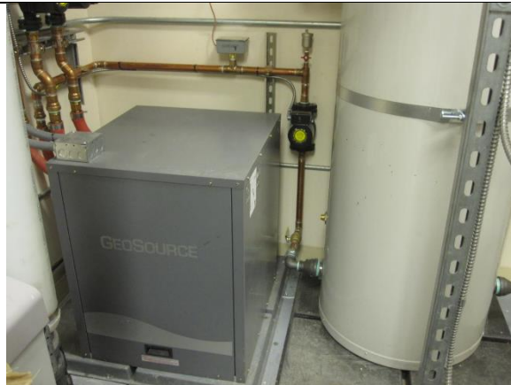
Installed 3 ton heat pump
